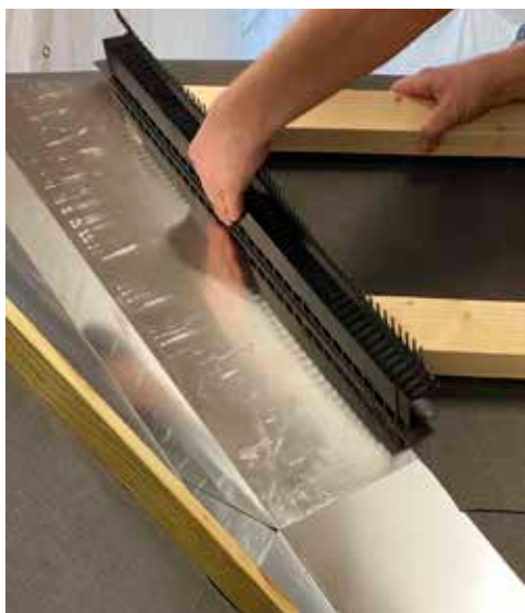
Clamp the first valley element tightly around the valley batten.
