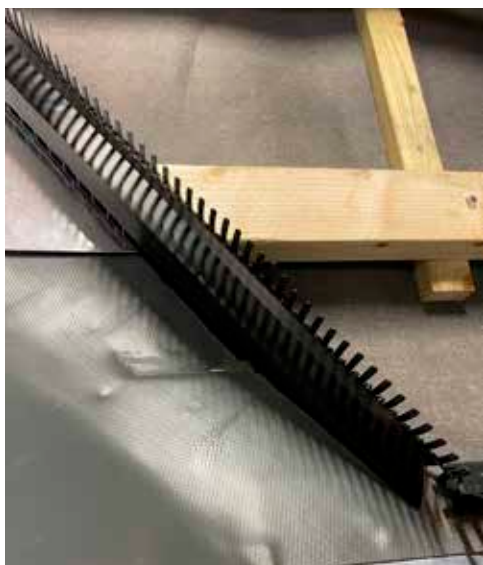
Finish with an element that is trimmed to fit the slope of the drip edge.
