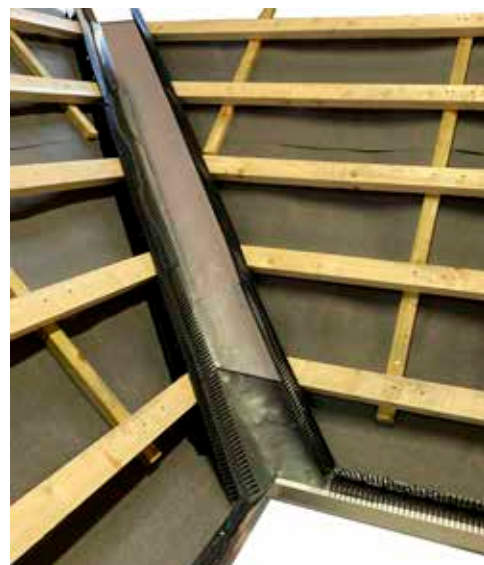
Valley elements installed and ready for laying roof tiles.
