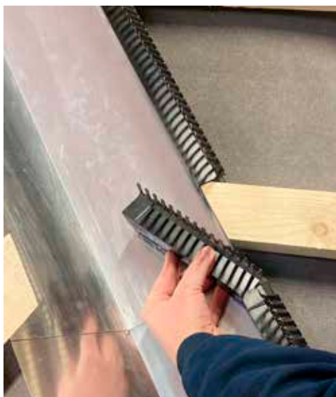
Any gaps should be covered with a cut piece of element.
