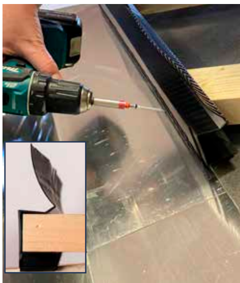
Fix with a screw in the valley batten from the side or from the top.
