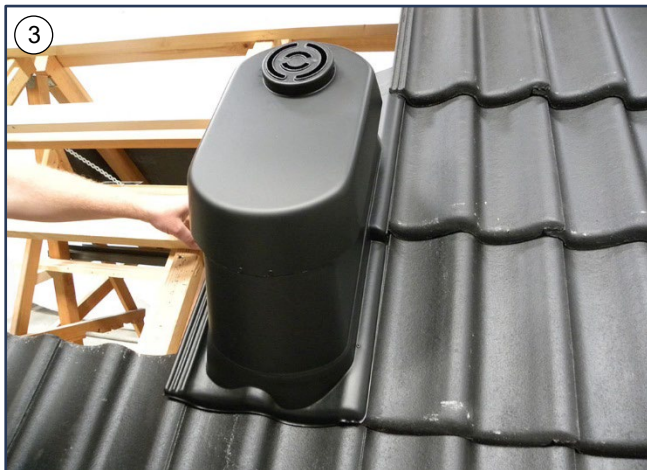
Outlet installed in roof construction.
