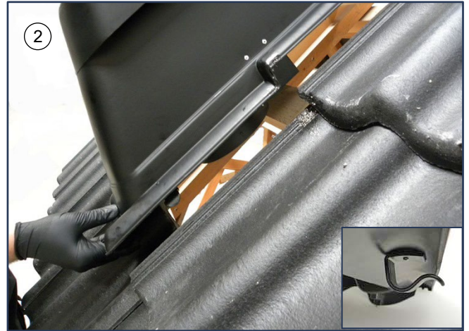
Outlet is installed like the roof tiles, fixed with clamp
