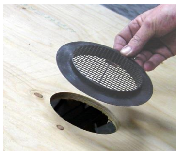
Apply suitable sealant on the UV2003 and fix to the board.
